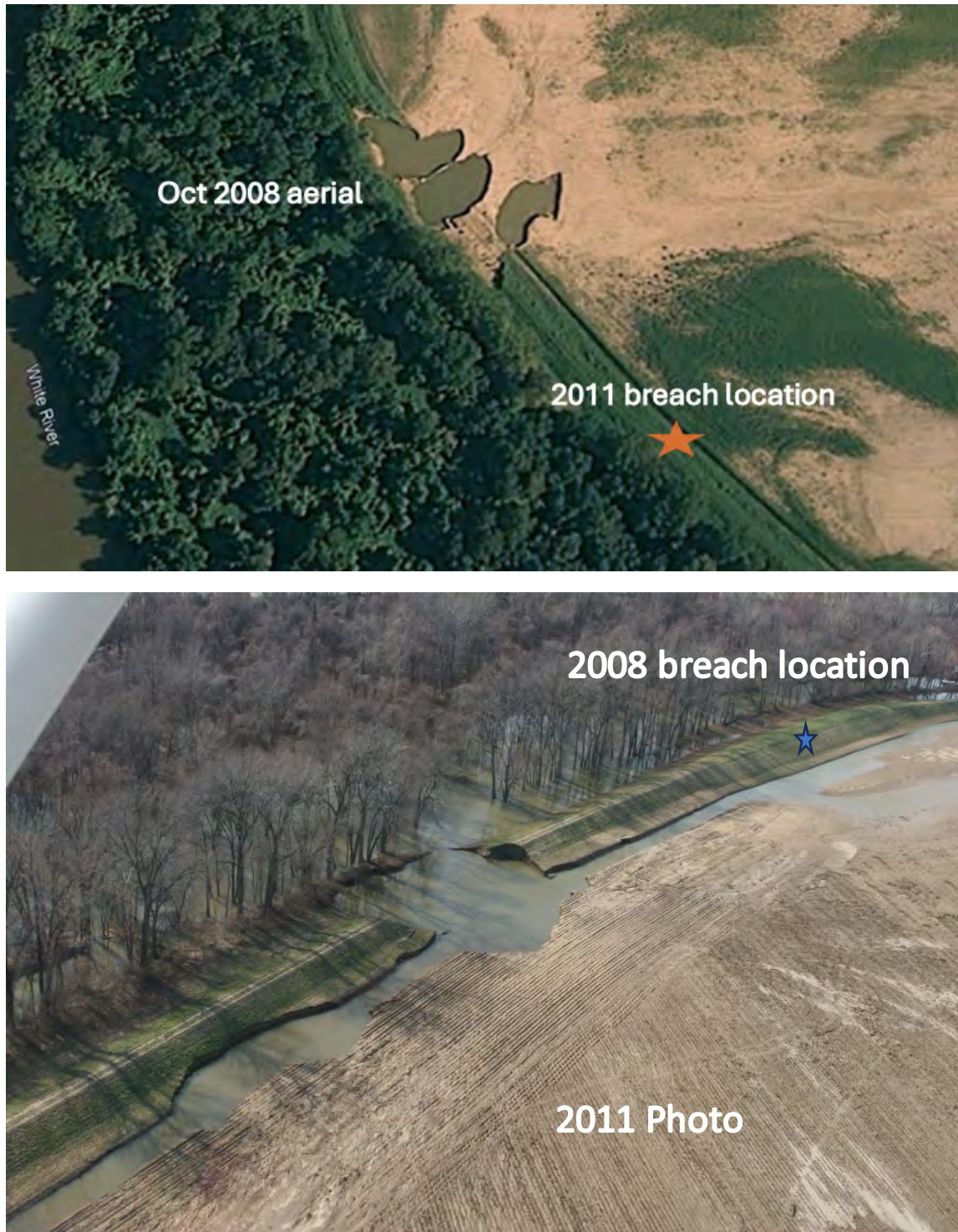
Figure 35. Levee Unit 8 2008 and 2011 Breaches
