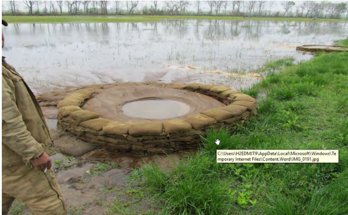
Figure 38. First and Second Boil During Flood
