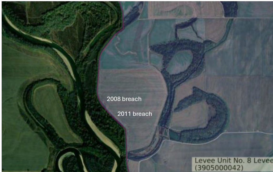
Figure 36. Levee Alignment at Breach Locations
