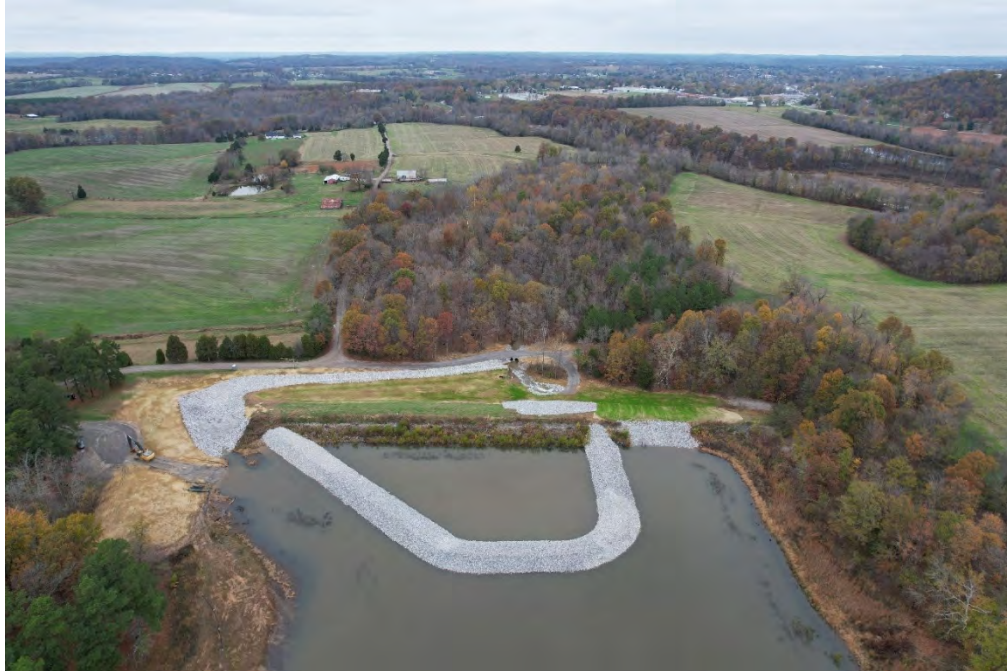
Figure 10. Completed IRRM Project Looking Downstream
