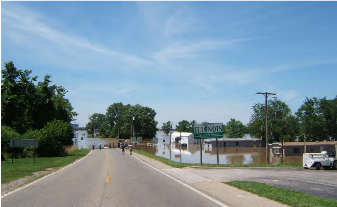
Figure 16. Photo of Illinois Flooding within the Russell Allison Leveed Area
