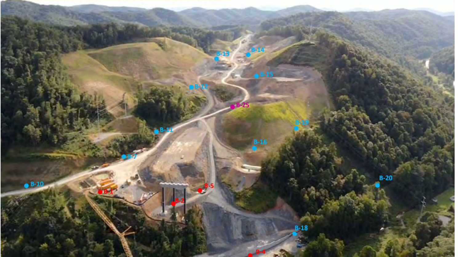
Locations of Currently installed Inclinerometers and Piezometers
