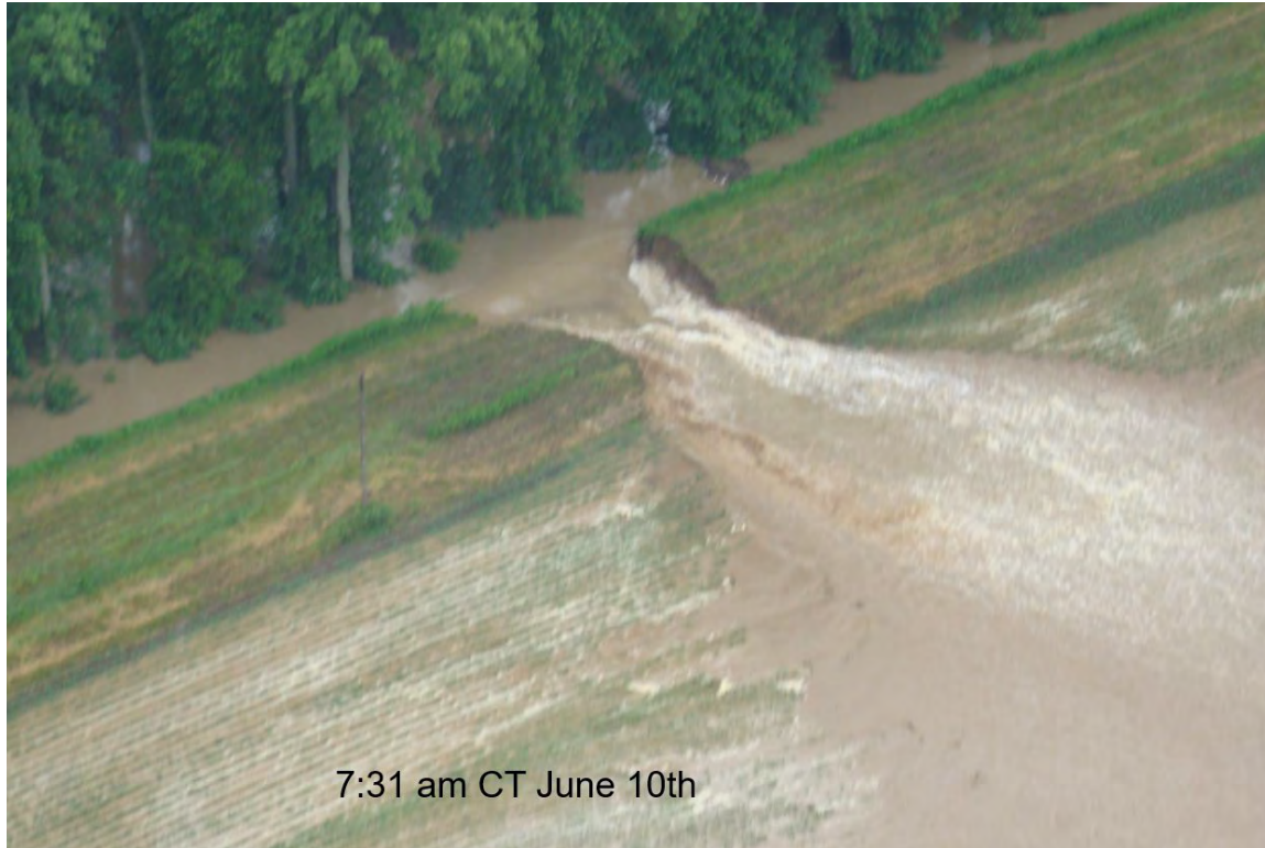
Figure 12. Russell Allison Levee Breach
