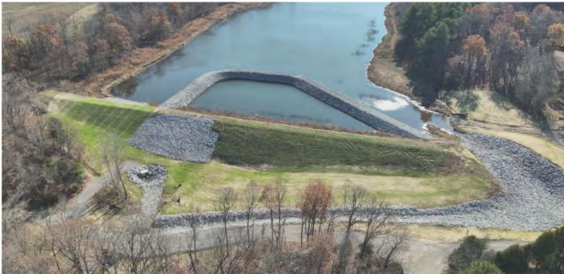
Figure 11. Completed IRRM Project Looking Upstream
