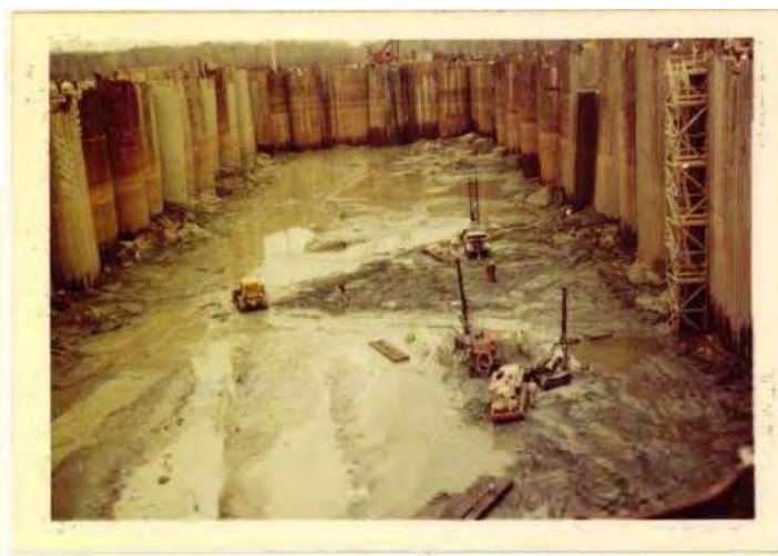
Slide Photograph No. 7, 25 Feb 71 - Cofferdam interior from Cell #15 looking toward Ky. Core drill on C-8-4, Air Track drilling gatebay 6 pre-split holes.
