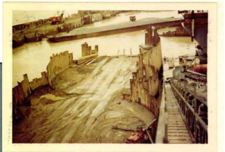
Slide Photograph No. 10, 26 Feb 71 - View of Cells #20 and #21 with connector arc, taken from concrete mixer barge, viewed toward Ky. Note aggregate barge inside cofferdam.
