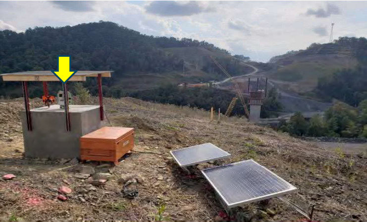
Photo 4: RTS #2 used to measure displacements of prisms above ground
