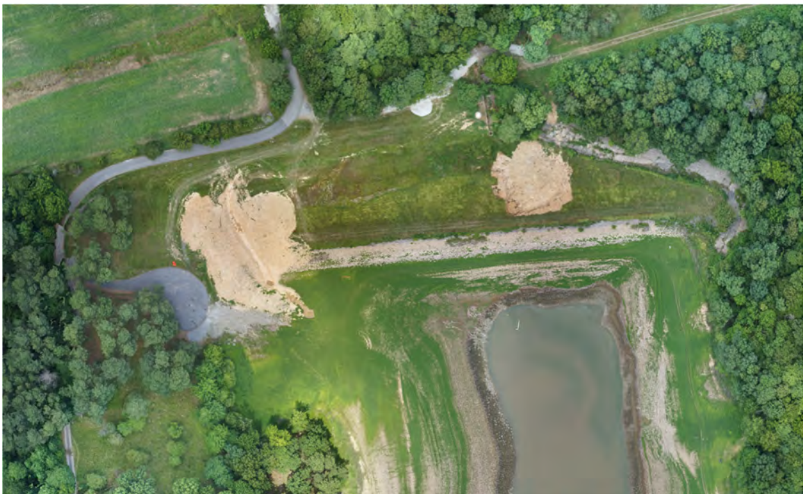
Figure 7. Post Failure Aerial from June 2022
