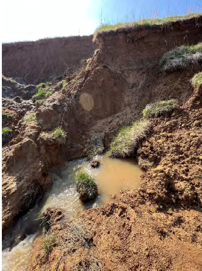
Figure 8. Seepage in Excavated Area (March 2023)
