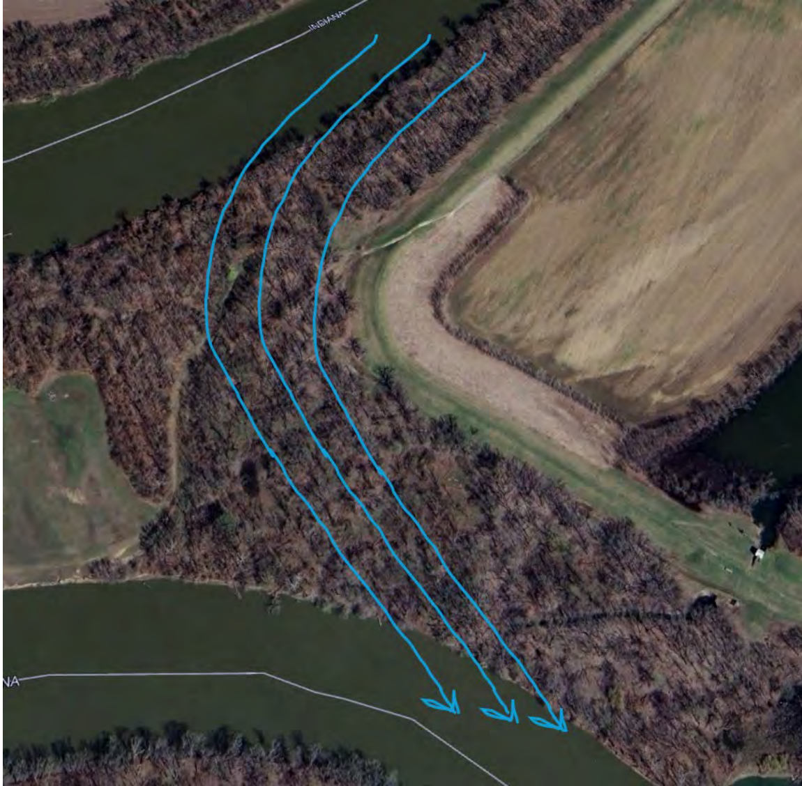
Figure 23. High Water Flow Path Adjacent Levee
