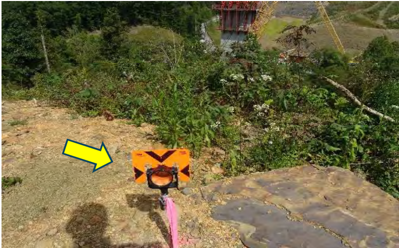
Photo 5: Typical prism used to monitor ground surface deformations
