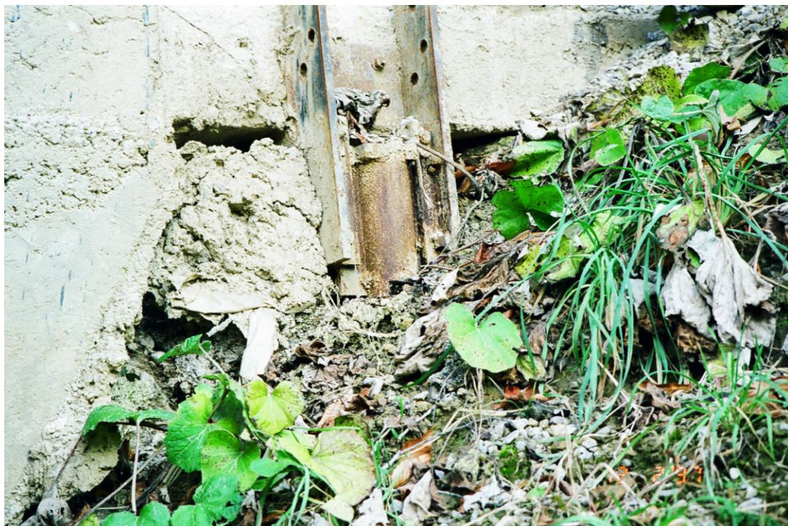
Fig. 6. West wall being underpinned with an Atlas pier.
