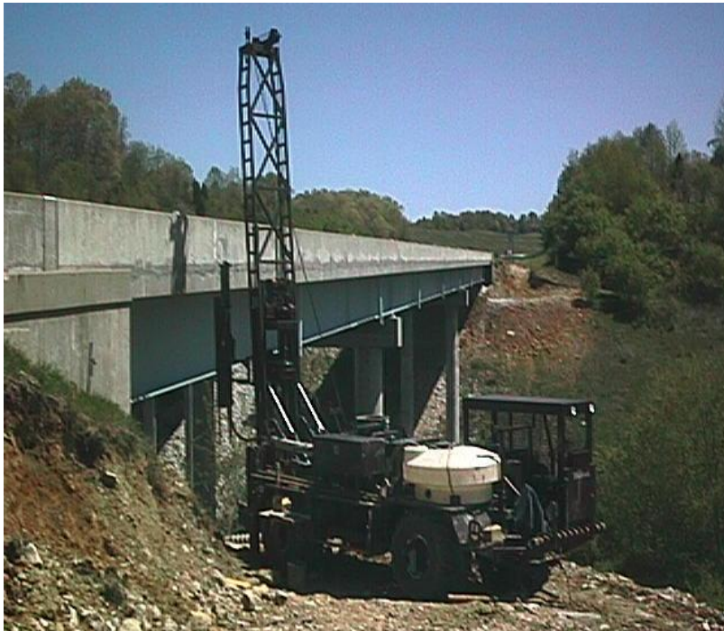
Fig. 12. Drilling vertical hole in west abutment slope to install coaxial cable.
