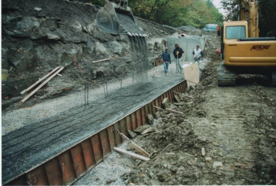
Fig. 16. The start of the geogrid reinforced wall
