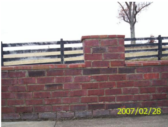
Fig. 22. Pre-blast photo of brick planter.
