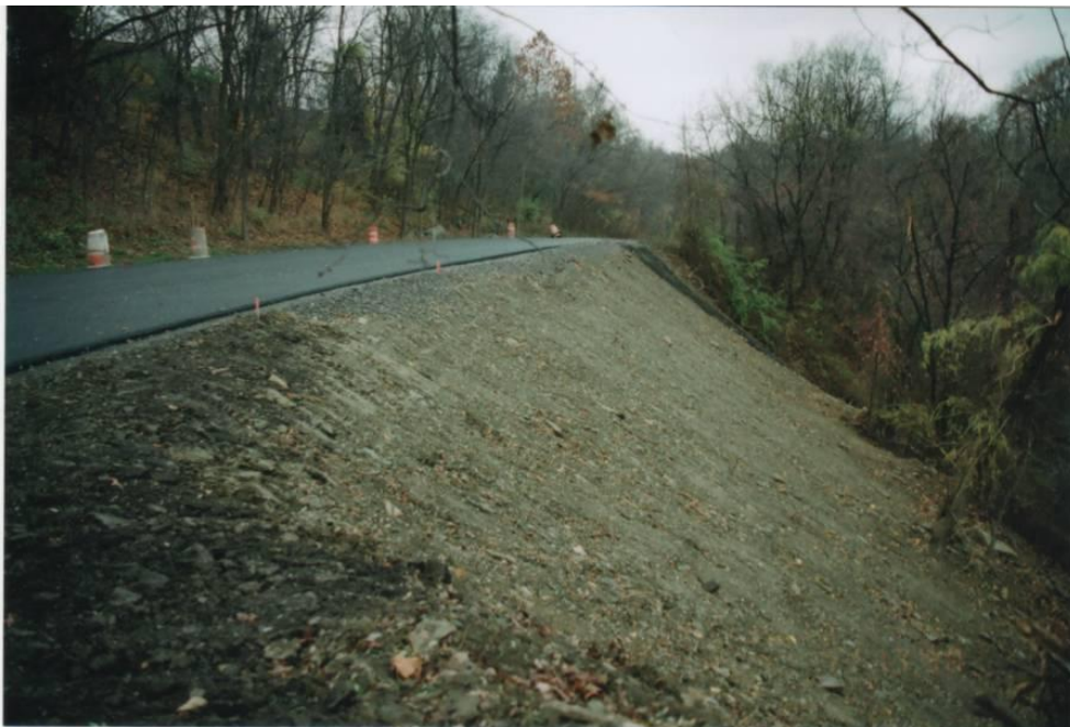
Fig. 19. The completed repair
