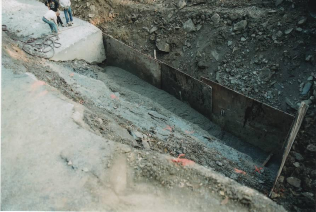
Fig. 14. Extension of concrete block foundation in area of sloping rock
