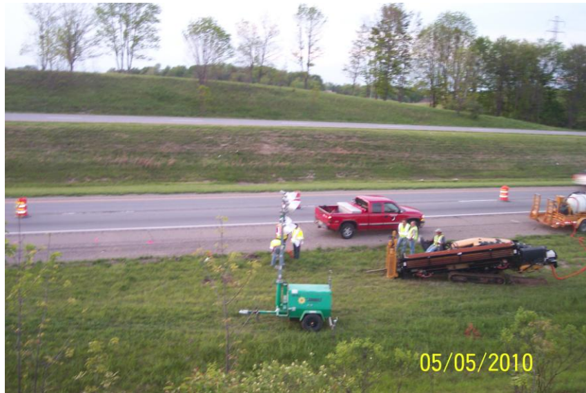
Fig. 8. Horizontal direction drilling below eastbound lanes of I-70
