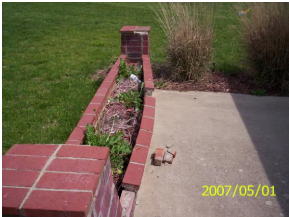
Fig. 23. Post-blast photo of brick planter.
