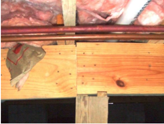
Fig. 7. View of wood beam support in crawl space.
