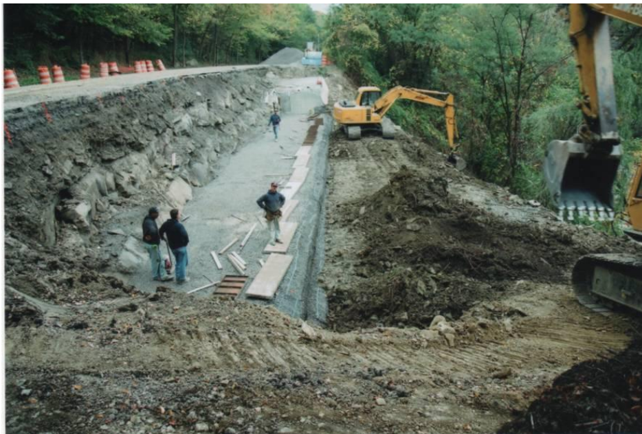
Fig. 17. The geogrid reinforced wall at mid height
