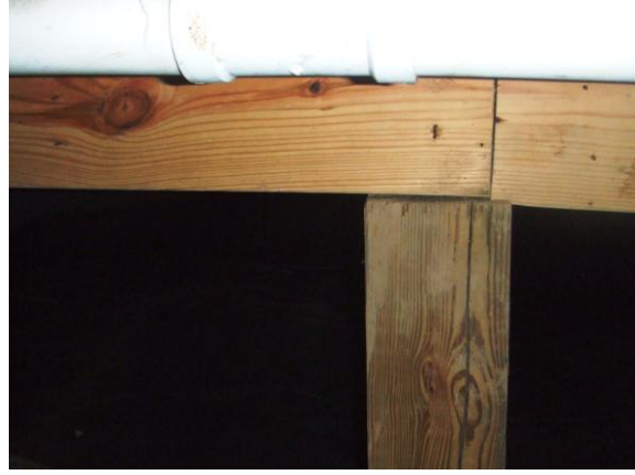
Fig. 8. View of wood beam support in crawl space.
