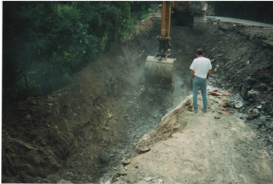
Fig. 10. Excavation at the north end of the slope repair
