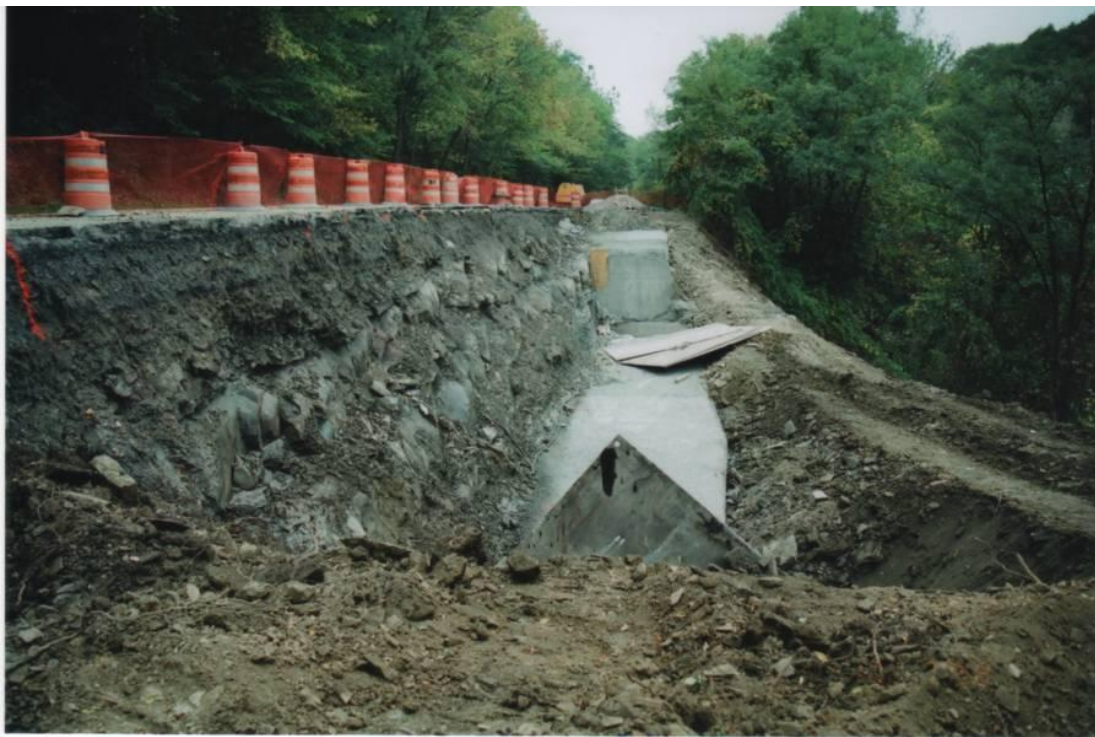
Fig. 15. Concrete block foundation looking south to north
