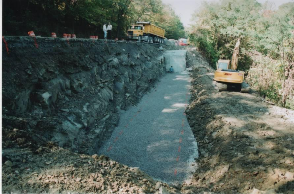
Fig. 18. The geogrid reinforced slope looking south to north
