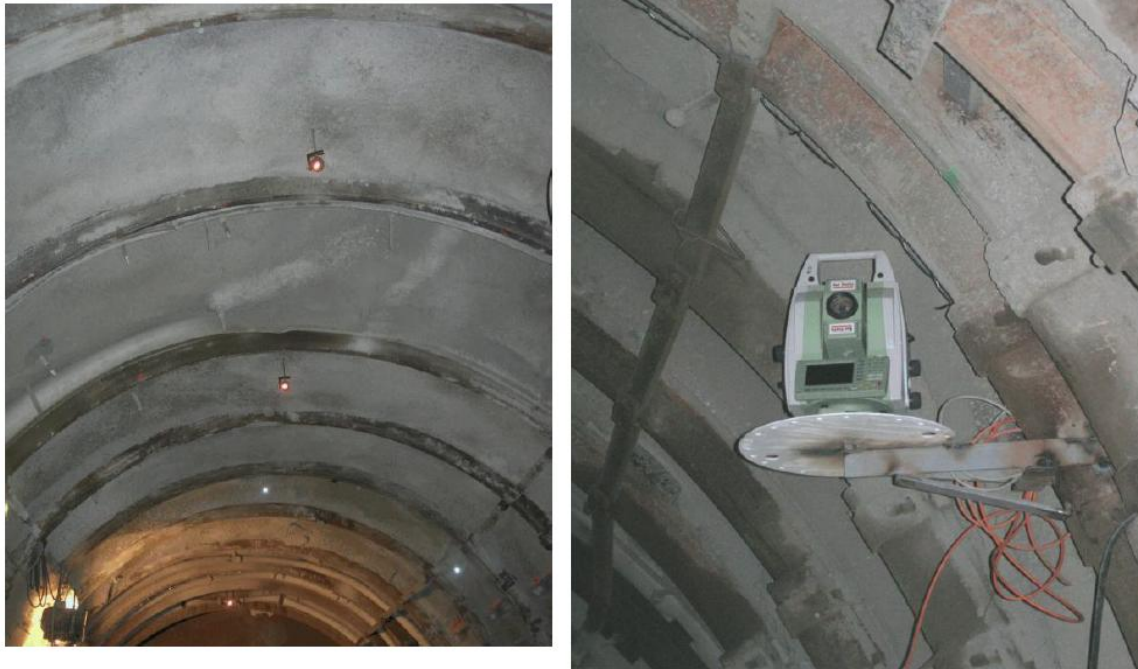
Fig. 6. AMTS and targets inside the gallery
