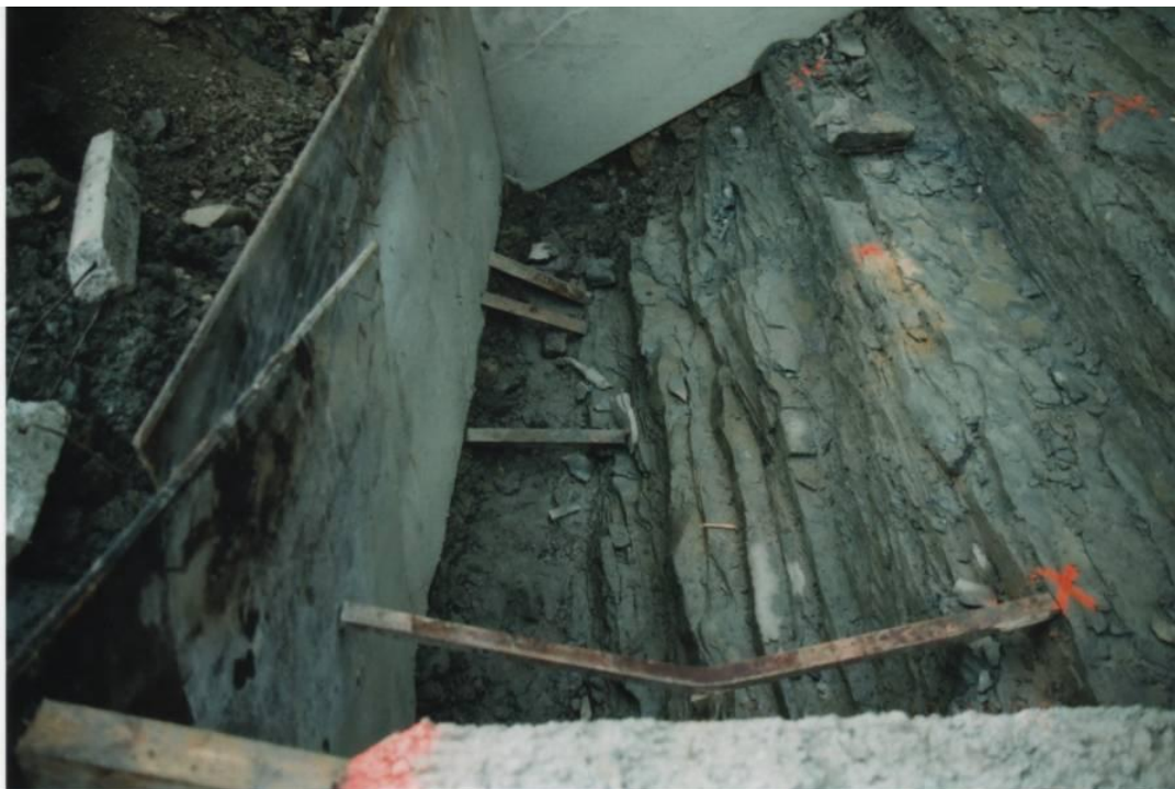
Fig. 13. Form work in area of sloping rock
