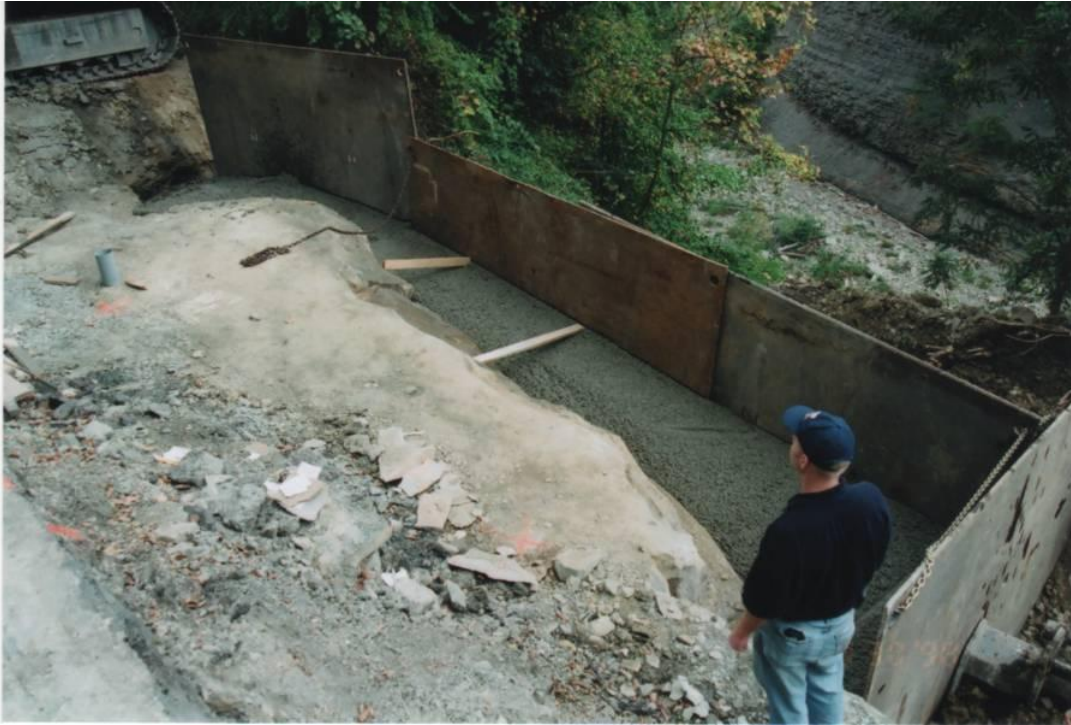
Fig. 12. Southward extension of the concrete foundation for the geogrid wall
