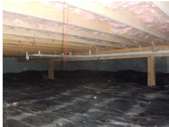
Fig. 6. View of wood beam in crawl space.
