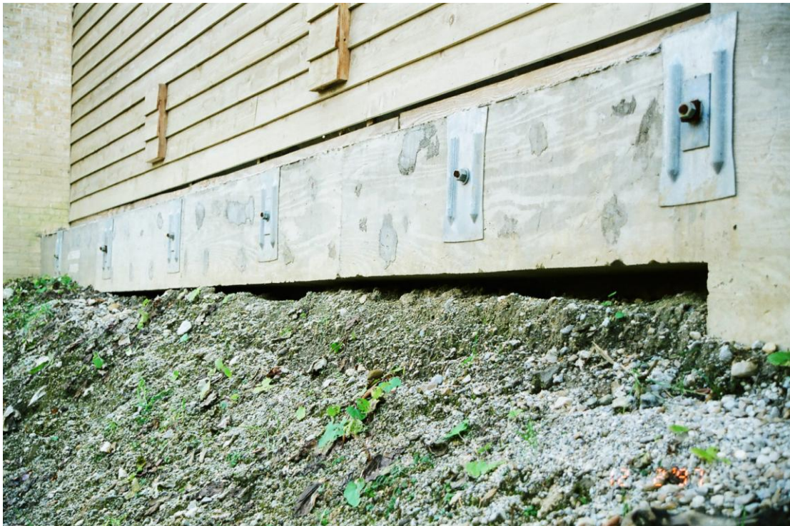
Fig. 5. Underpinned and tied back downhill foundation wall.
