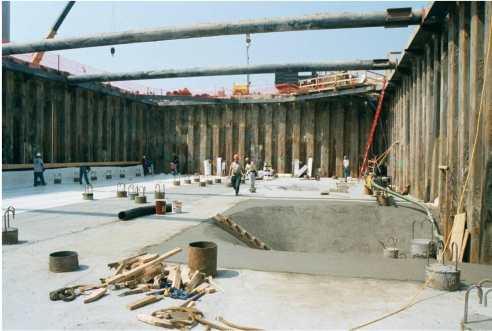
Fig. 5. Pump house and cofferdam with effective groundwater seal
