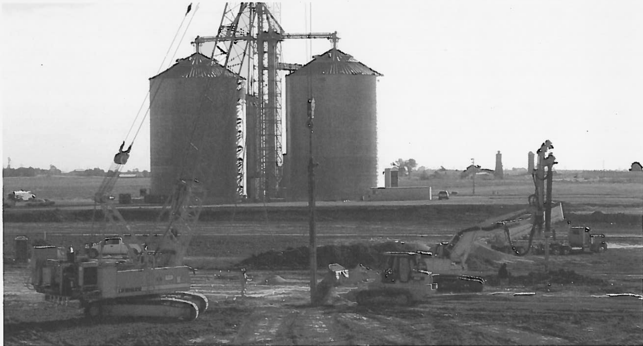
FIGURE 4 Crane, loader, and pre-drill rig being used to install aggregate piers.
