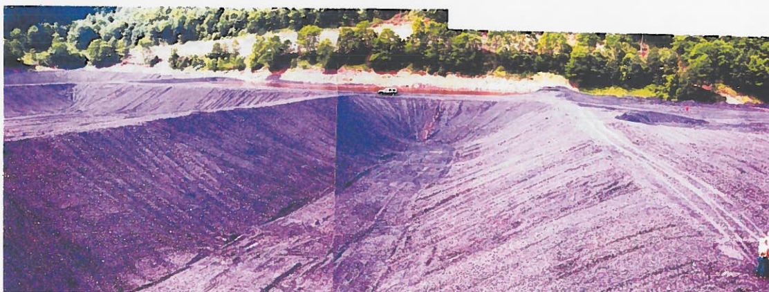
FIGURE 5 CASE HISTORY NO. 2 EXCAVATED FINE REFUSE CELLS
