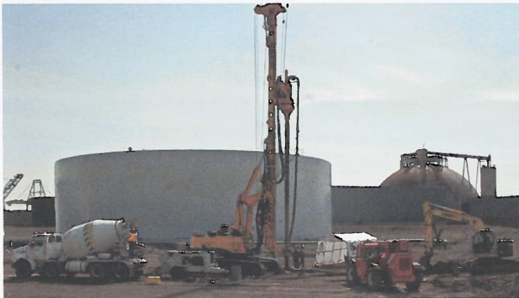
FIGURE 7 Installation of the CMCs in Quebec City.
