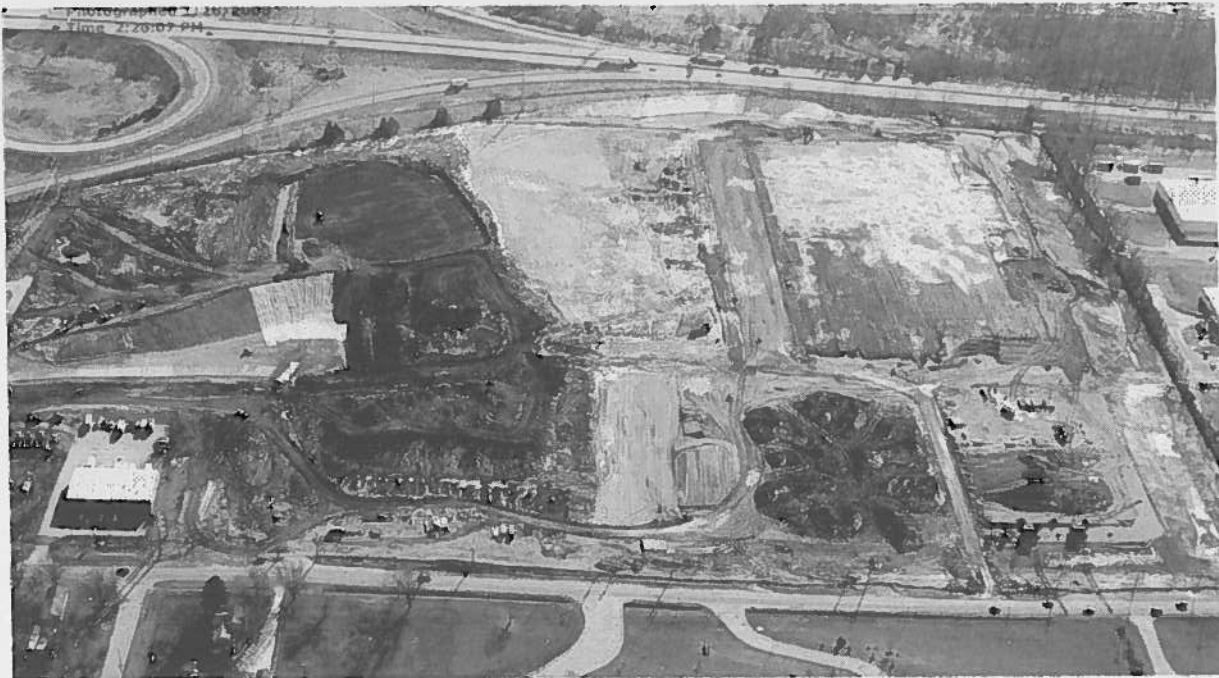
Figure 5. Site Development Activities About Mid-way through Project – looking south
