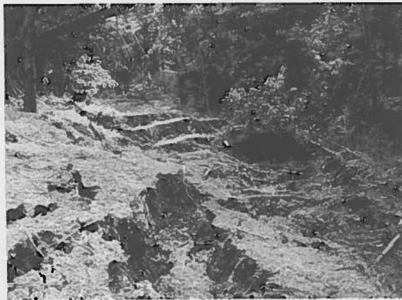
Figure 9. Surface expression of progressive failure
