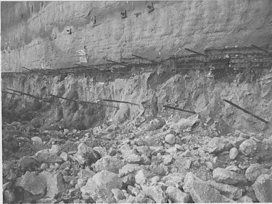
FIGURE 9 – Block 76 Jet Grout Wall South Temple Street
