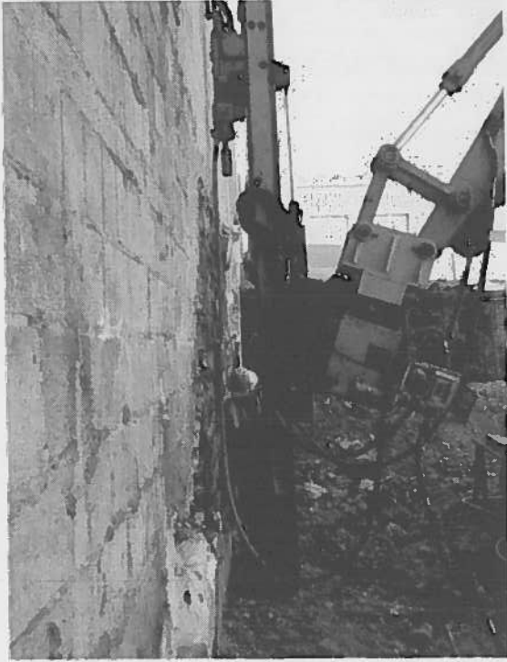
FIGURE 7 – Block 76 Marriott Hotel Underpinning Micropile Installation
