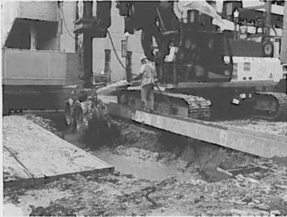
Figure 10. CSM Rig at North Shore
