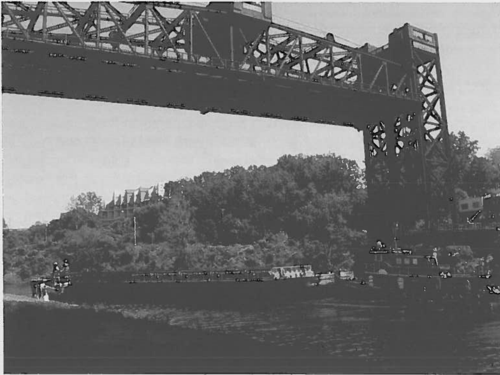
Figure 6. - Columbus Road Lift Bridge
