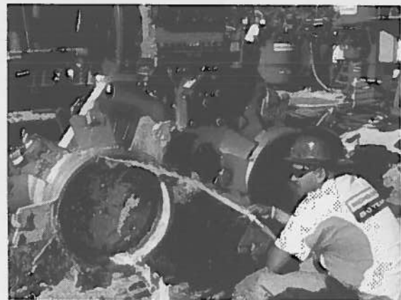
Figure 9. Cutting/Mixing Drums of CSM
