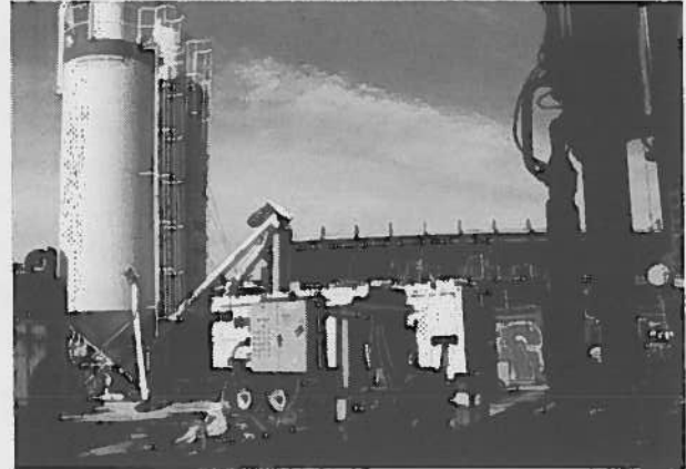
Figure 11. Grout Plant at North Shore
