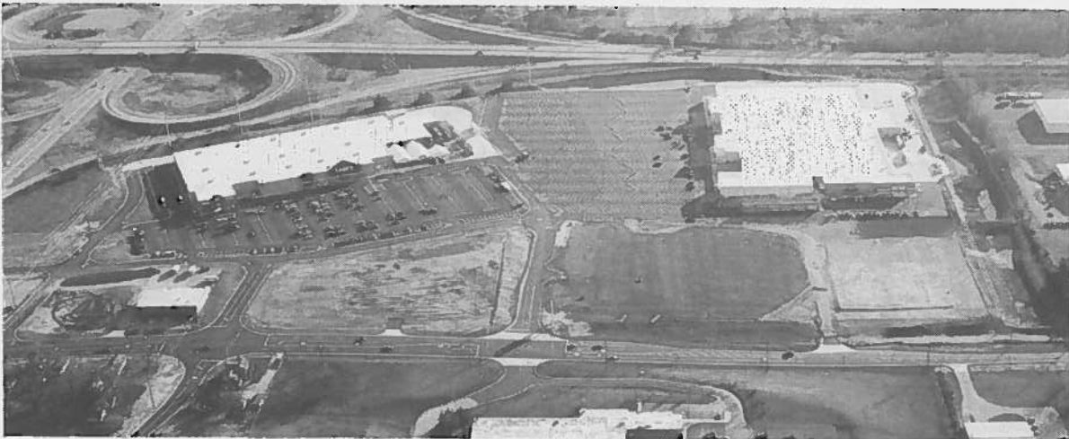
Figure 6. Site Development Activities Substantially Complete, looking south
