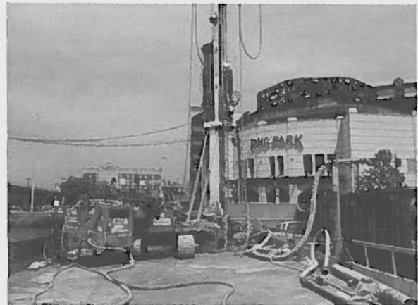
Figure 5. Spoil Management at Launch Pit
