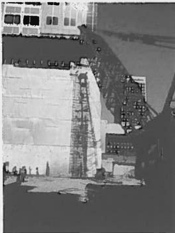
FIGURE 11 – Block 76 Diaphragm Wall at Gateway Tower Cage Placement
