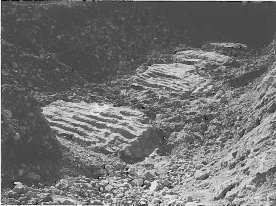
FIGURE 8 – Block 76 Jet Grout Test Columns – Initial Excavation
