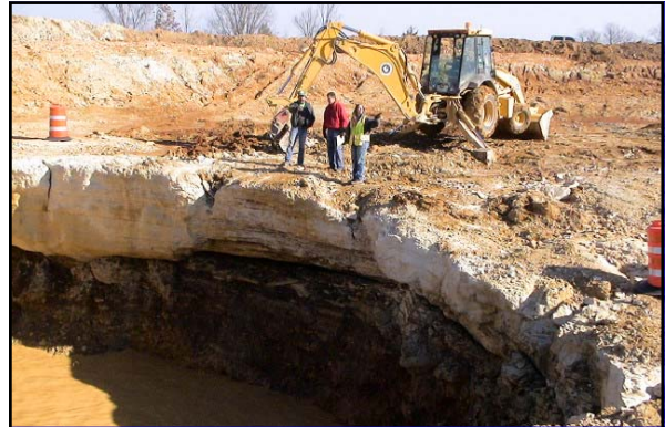
The upper 5 ft of rock was jointed but not extensively fractured; the lower 10 ft (to water line) was extensively fractured and could be readily dislodged with a shovel.
