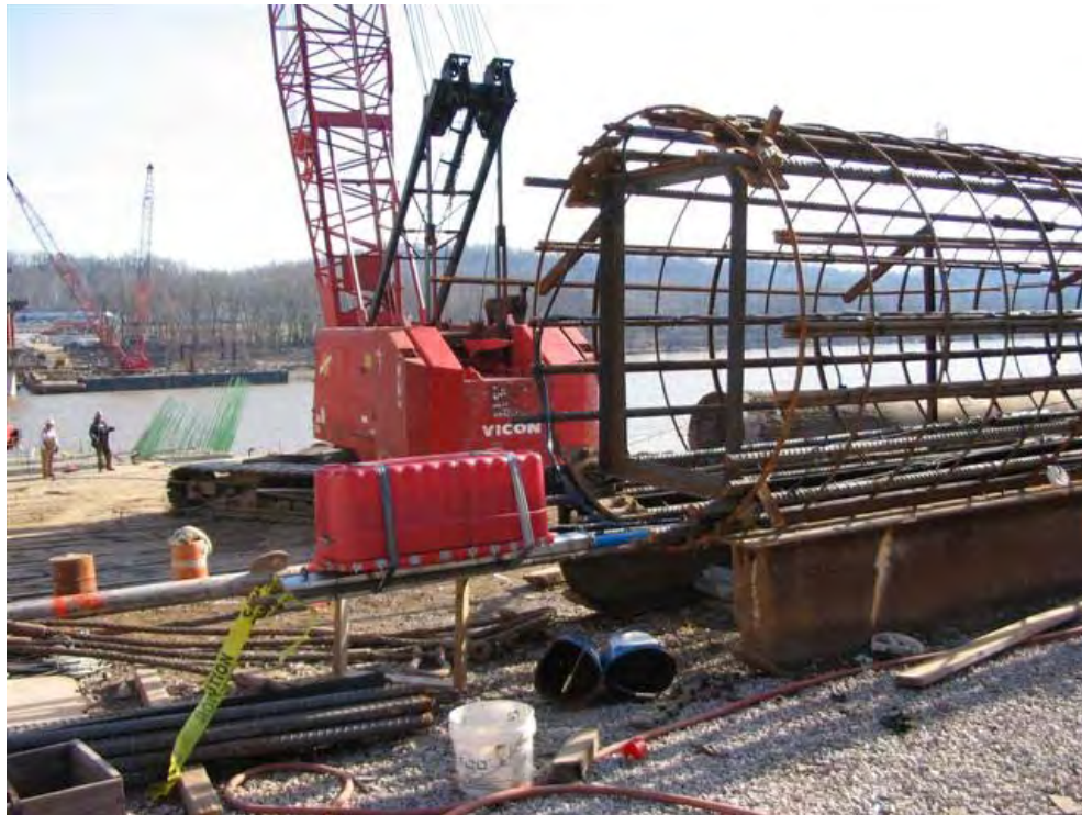
Figure 11. Reinforcing Steel Cage Being Prepared
