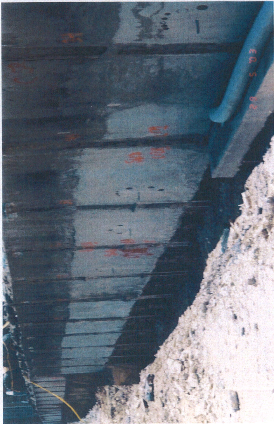
FIG. 2 TIED-BACK SOLDIER PILE WALL SHOWING CIP CONCRETE LAGGING
