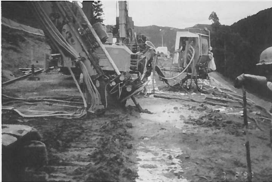
Figure 6. Drilling machine for micropile installation.
