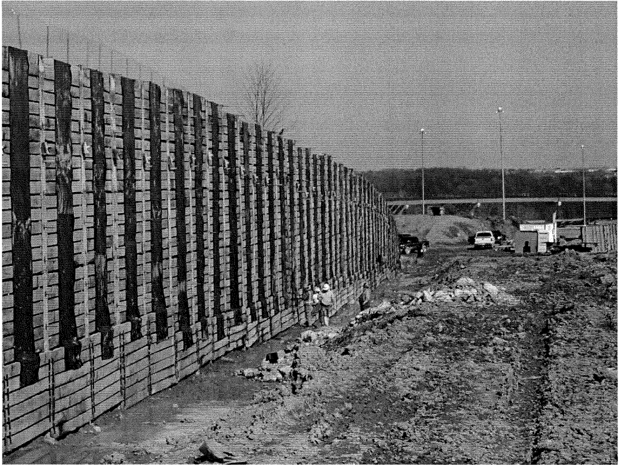
Figure 3 – Placing drainage mats to full temporary height.
