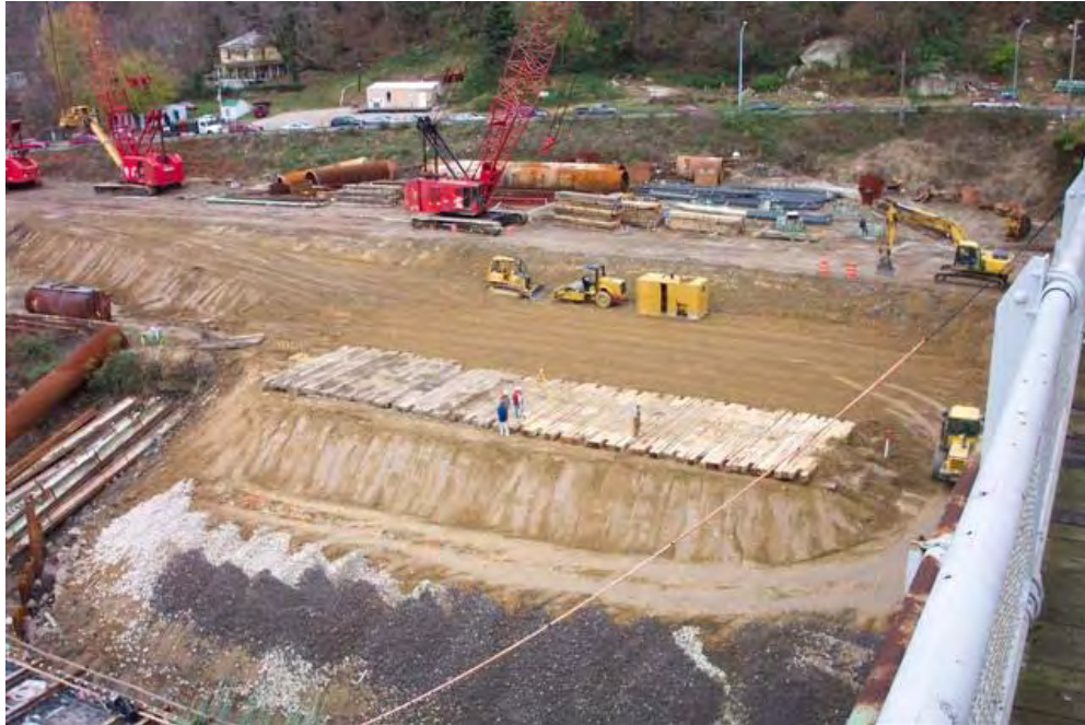
Figure 10. Work Pad Being Prepared for Stabilization Shaft Installation
