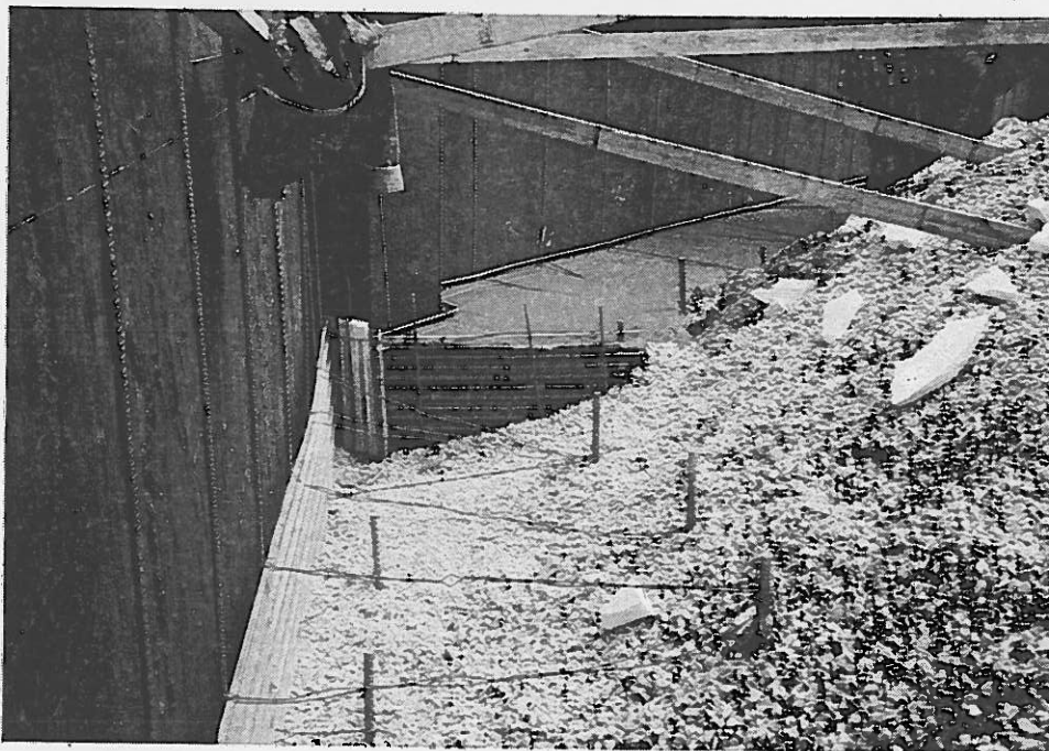
Figure 1. First Lift of CDF, Formwork, Soil Nails and Ties.
