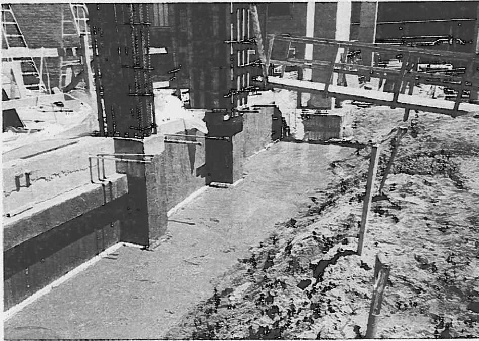
Figure 4. Completed CDF Fill With Foam Blocking At Wall
