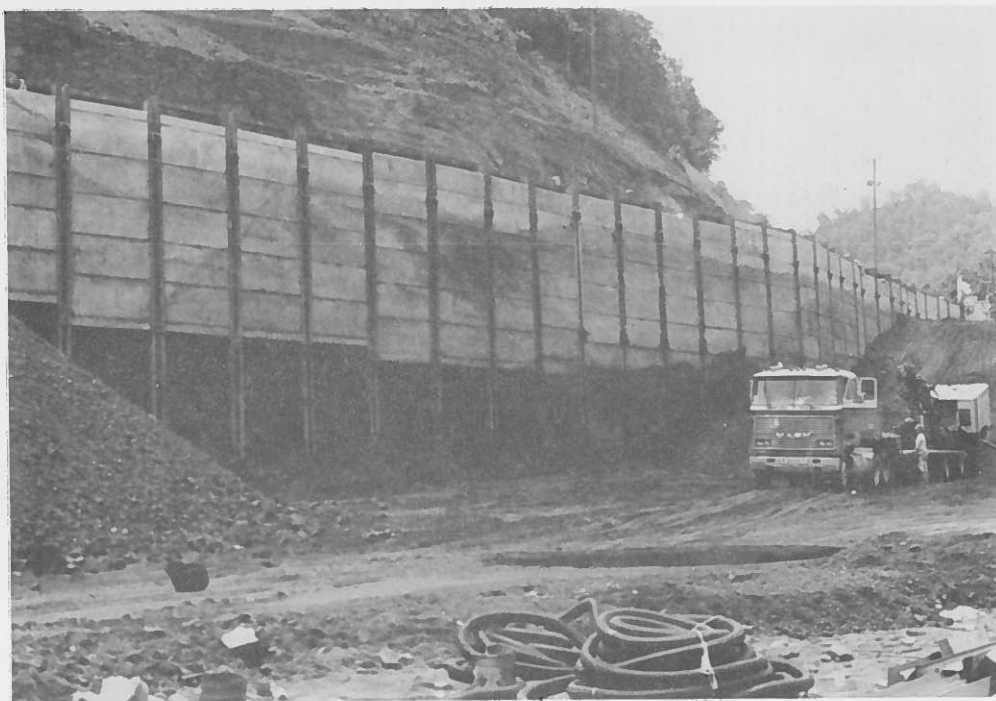
Figure 12. Photograph of completed tied-back coal dumping wall.
