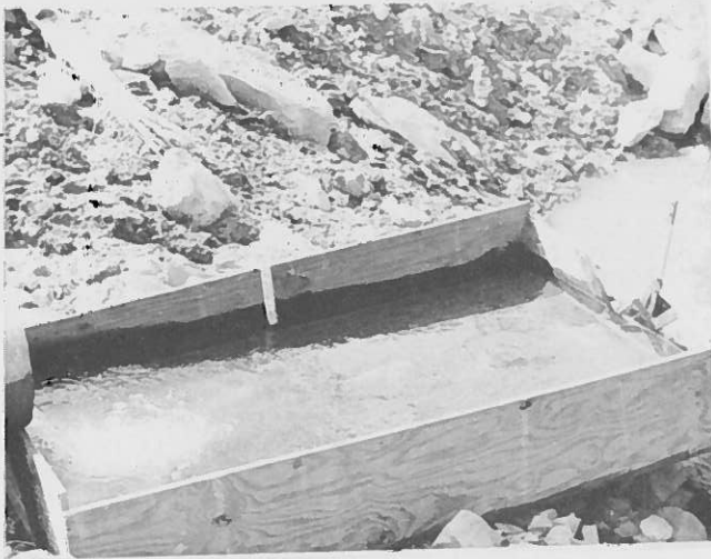
Figure 10. Weir for seepage control.
