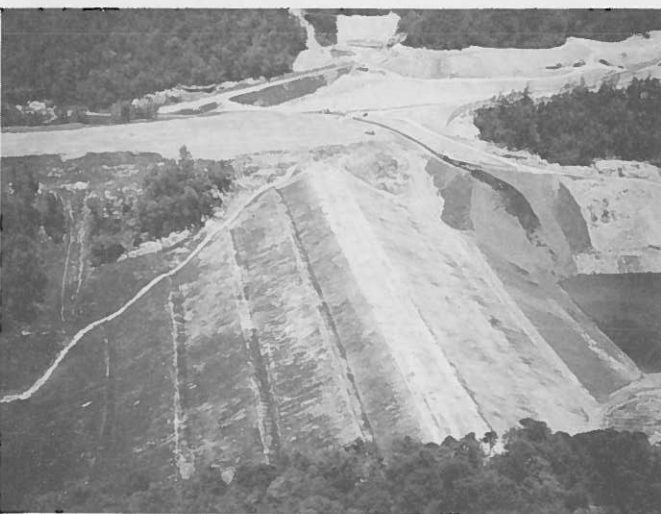
Figure 7. Case history No. 1 - Aerial View.
