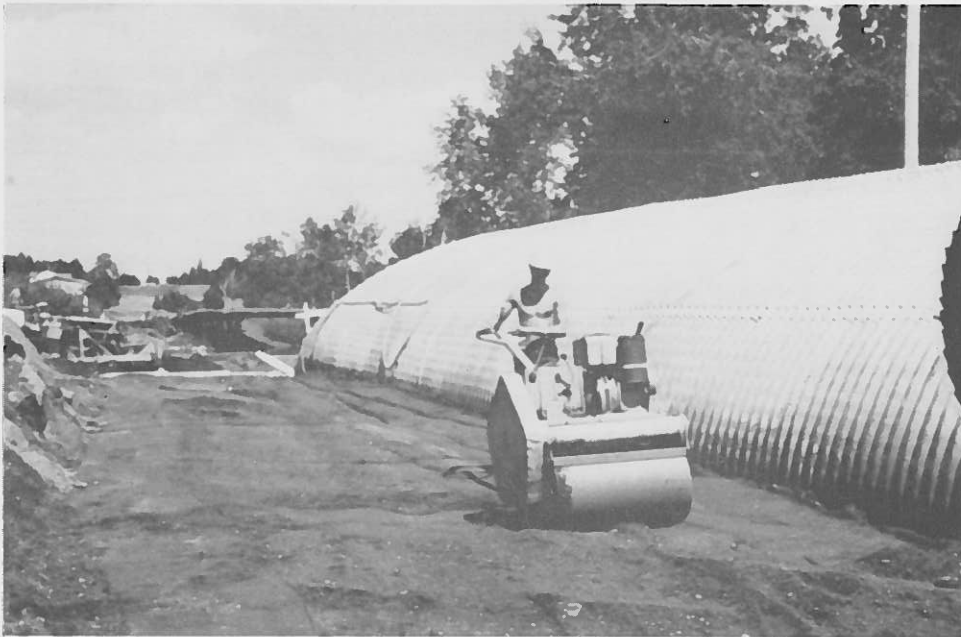
Figure 17. Compacting a Layer of Structural Backfill
