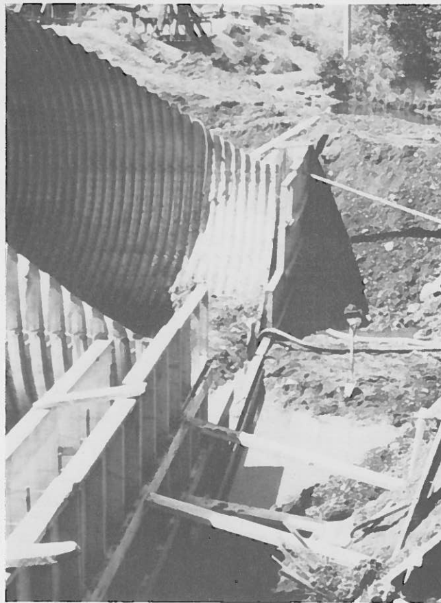
Figure 18. Constructing Concrete End Wall
