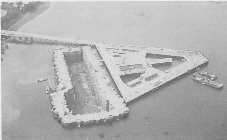
Figure 4 Aerial Photograph of Unwatered Cofferdam
