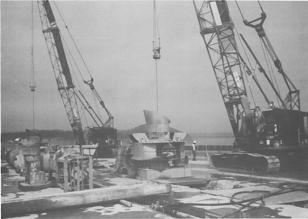
FIGURE 28. EXCAVATION WITH CLAMSHELL THROUGH TEMPORARY CASING. NOTE CASING DRIVER.
