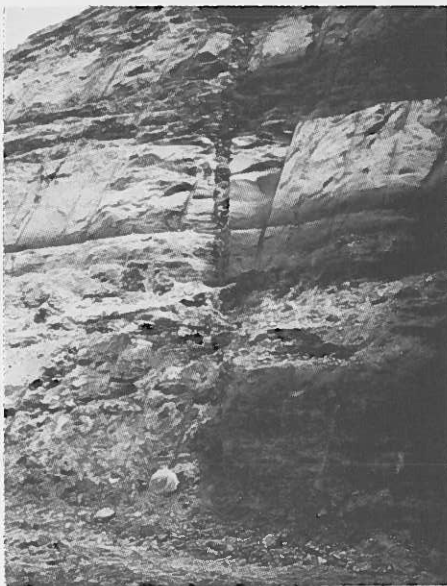
Fig. 4. Clay-filled joint, approximately 10 in. wide, in massive sandstone; abutment excavation for small dike in southern Indiana.
