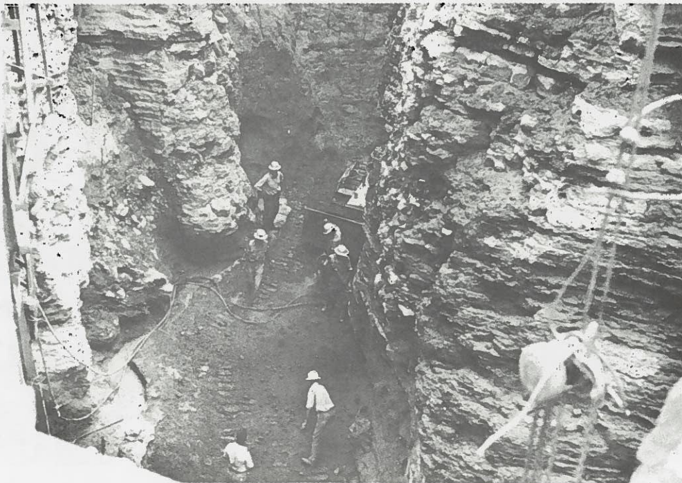
FIGURE 9. CUTOFF TRENCH AT CONCRETE STRUCTURE LOOKING LANDWARD.
