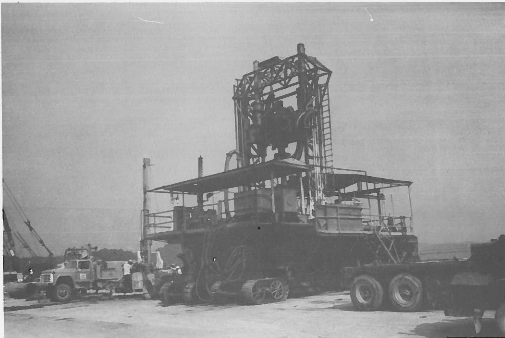
FIGURE 29. 36-INCH DIAMETER ROTARY DRILL WITH REVERSE CIRCULATION.
