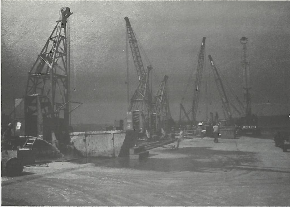
FIGURE 30. "WOLF CREEK" DRILL EXCAVATING SECONDARY ELEMENTS.
