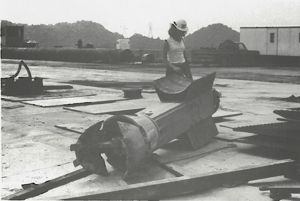
FIGURE 31. BI-CONCAVE CHISEL WITH SMALL CLAMSHELL FOR EXCAVATING SECONDARY ELEMENTS.
