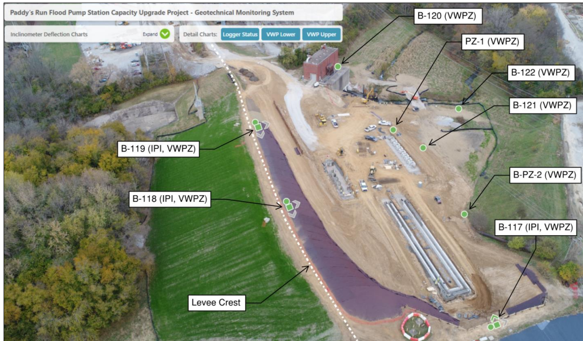
Figure 16: In-place slope inclinometer (IPI) and vibrating wire piezometer (VWPZ) locations.
