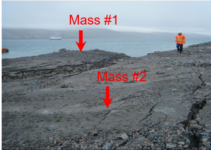
Figure 9. Photograph of slide masses #1 and #2 with the second slide mass developing without large displacement of the first slide mass (Note rockfall off the back of the first slide block into the gap between the two masses).
