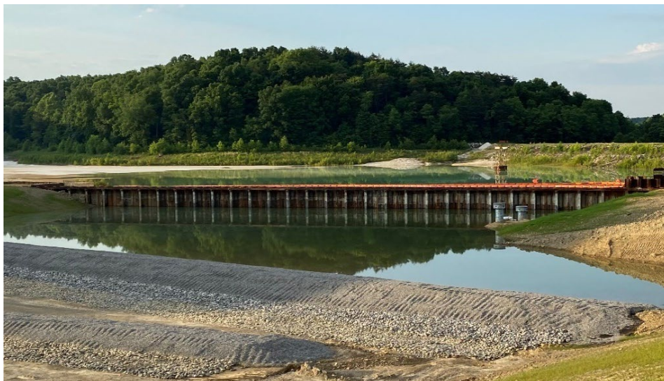
Fig. 7. Completed Sedimentation and Detention Pond 1B.
