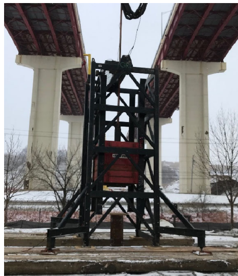
Figure 2: 28-Ton Drop Weight Hammer
