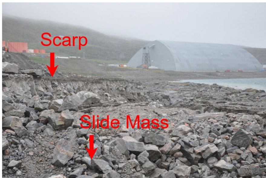
Figure 8. Almost vertical scarp through causeway of the last slide mass near the shore.
