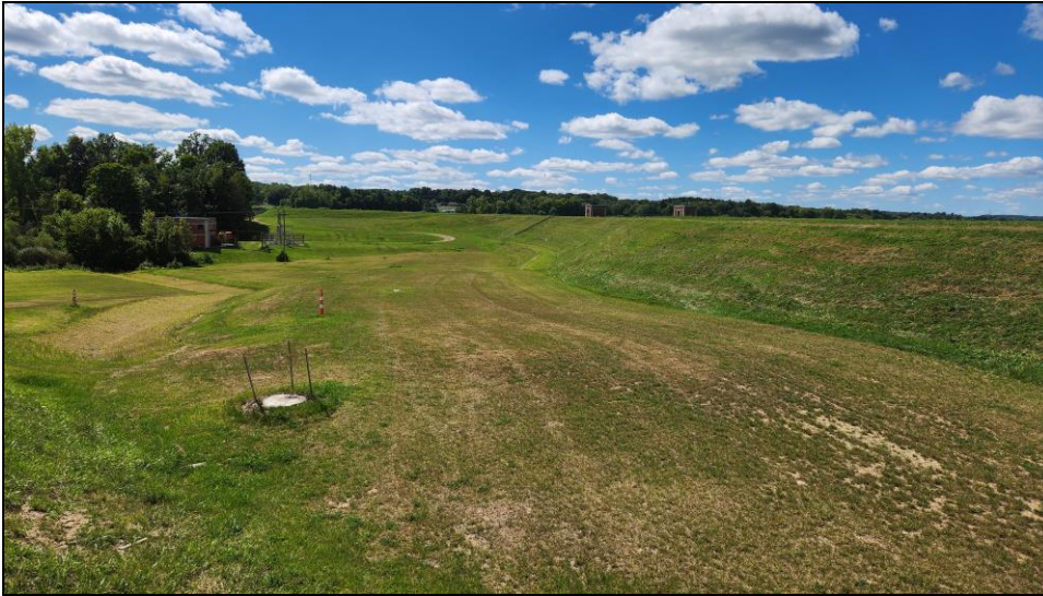
Fig. 12. Completed Construction of the Graded Filter Toe Berm
