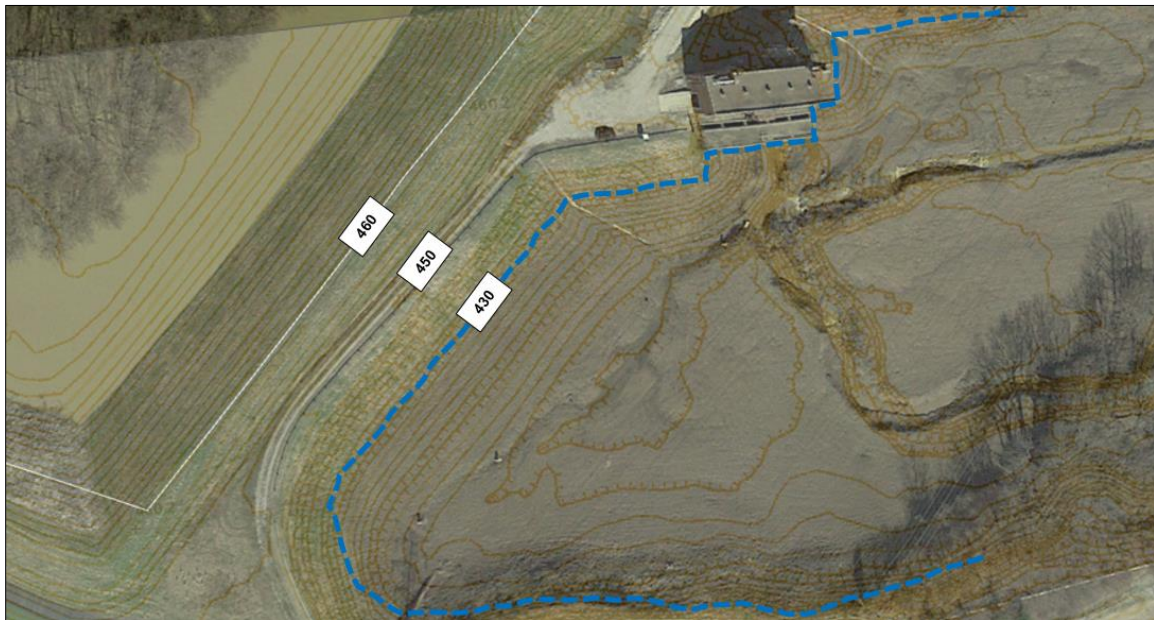
Figure 9: Aerial view of the ponding area on February 28, 2018, five days after the maximum P-1A reading of 429.36 feet (Google, 2018).
