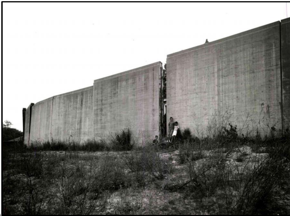
Figure 10: Floodwall Monoliths 43, 42, 41, 40, 39 and 38 (left to right)
