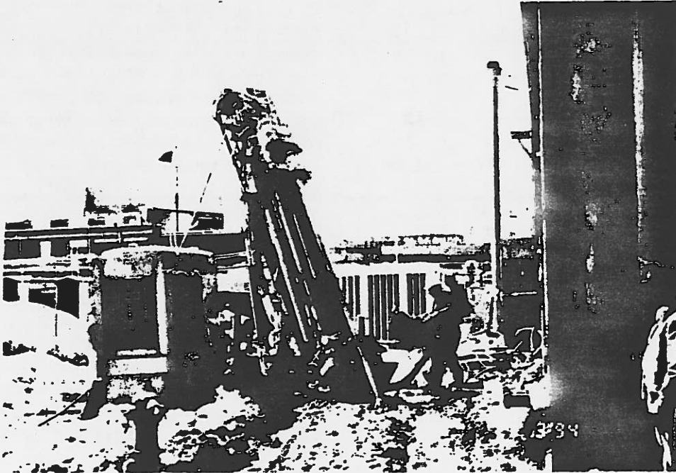
Figure 22. Jet pile installation
