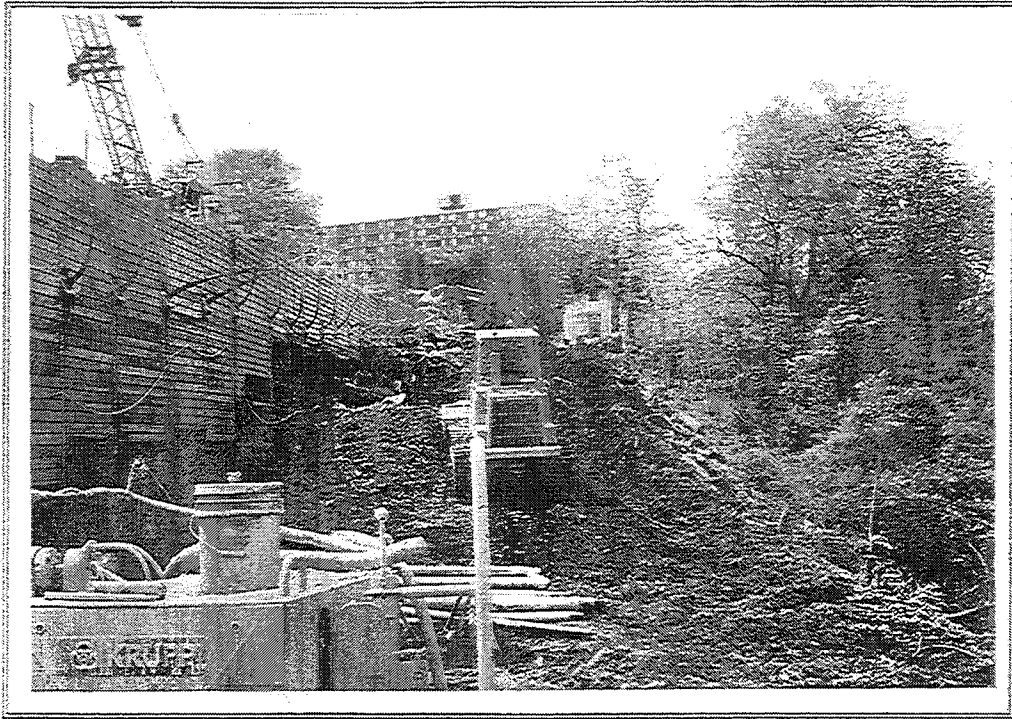
Figure 33. Downhill view of wall
