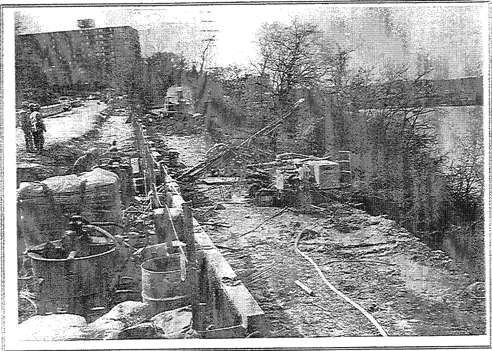
Figure 27. Installation of top row tieback anchors
