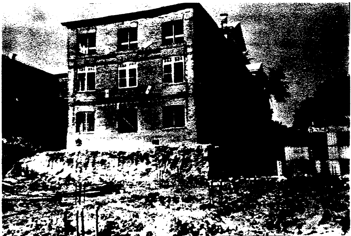
Photograph 2 - Excavation completed, the soilcrete wall is exposed.
