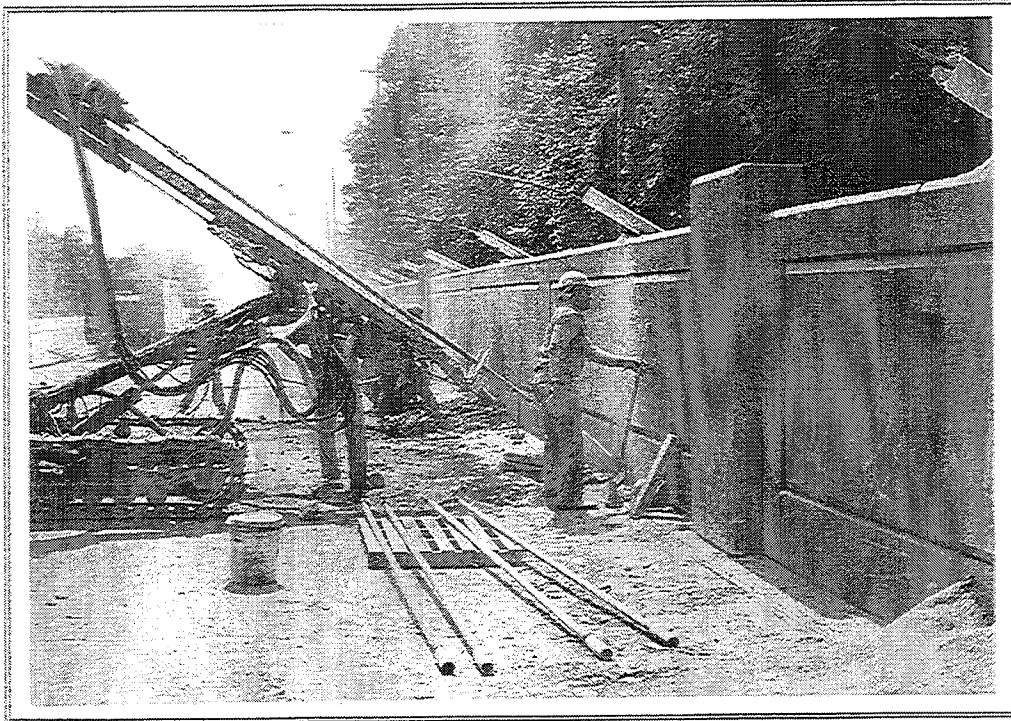
Figure 23. Installation of anchors in existing uphill wall
