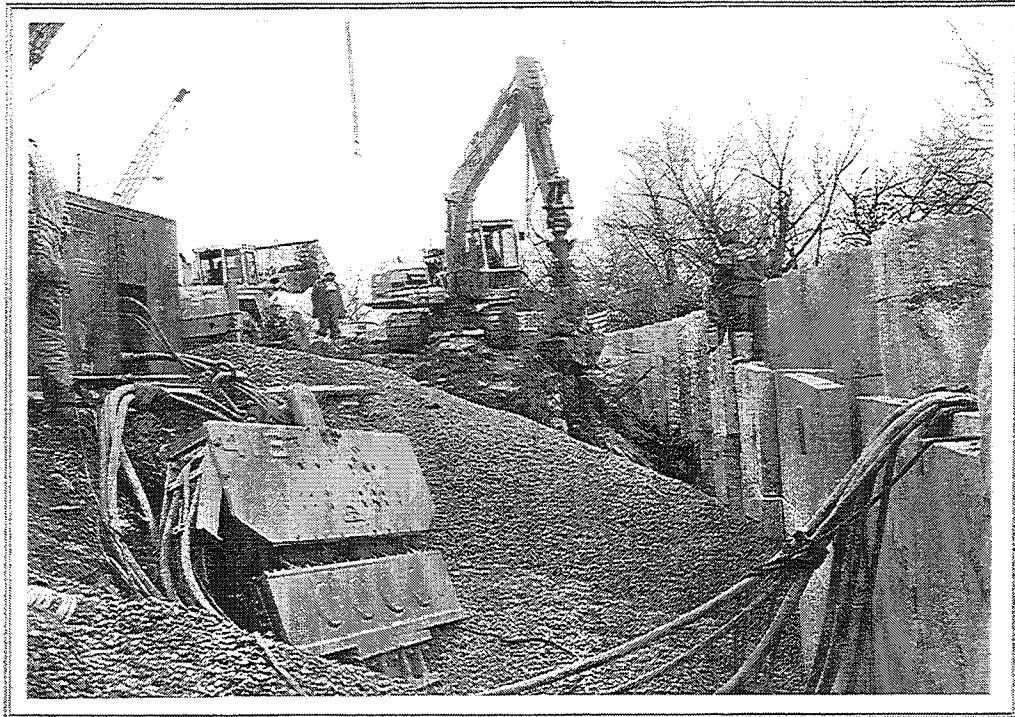
Figure 13. Excavation and backfilling
