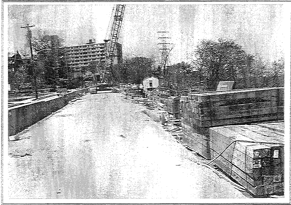
Figure 25. Traffic lane used as working bench
