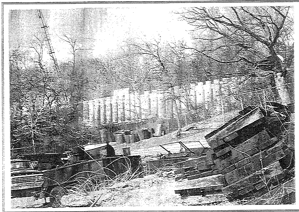
Figure 20. Downhill view of wall
