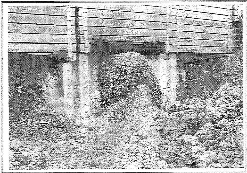
Figure 30. Soldier beams, lagging, studs, and drainage material
