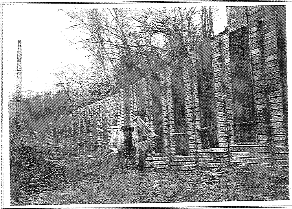
Figure 7. Placement of drainage material
