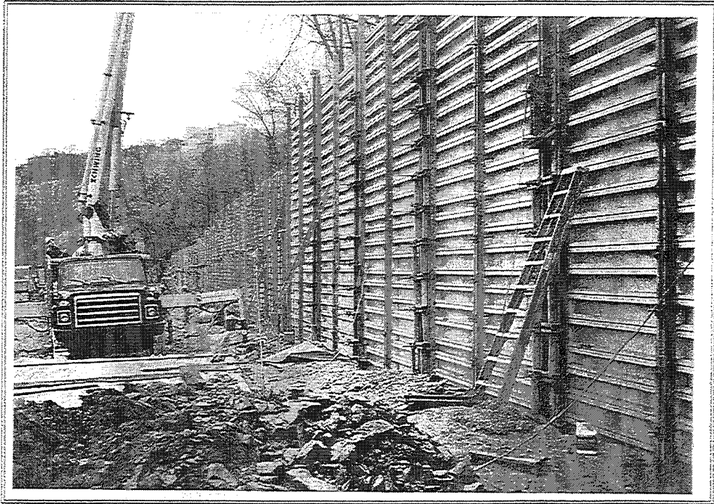
Figure 9. Facing wall gang forms
