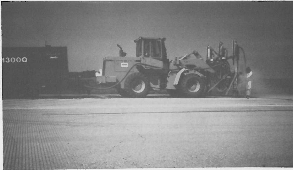
FIGURE 7 Rotary percussion drill unit with 3100 cfm compression trailer.
