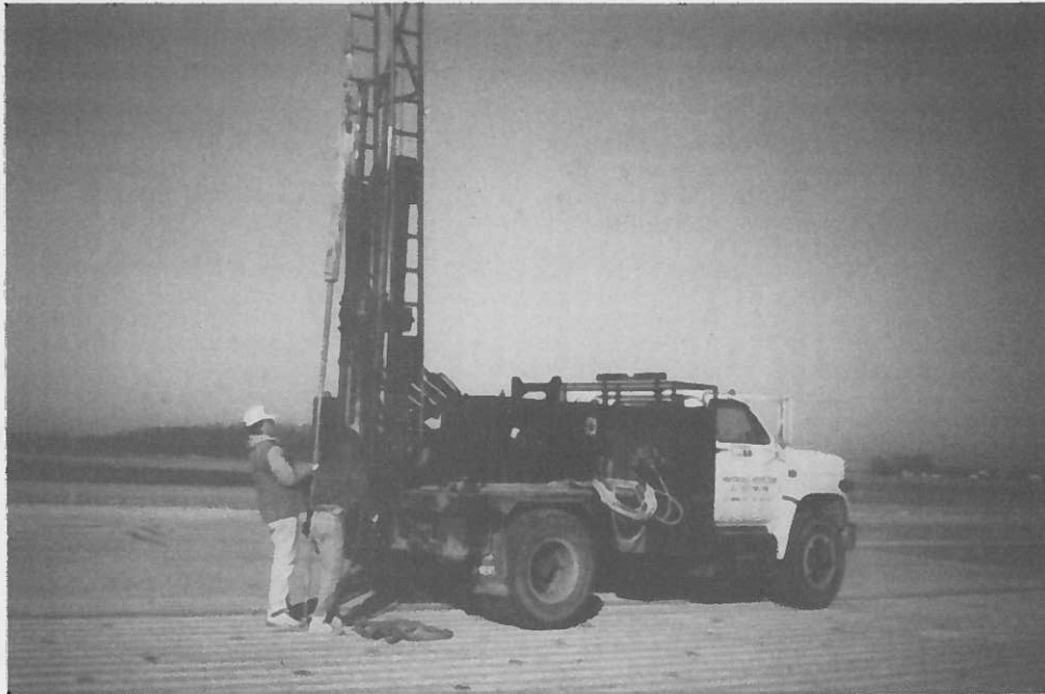
FIGURE 2 Obtaining pavement and soil samples.
