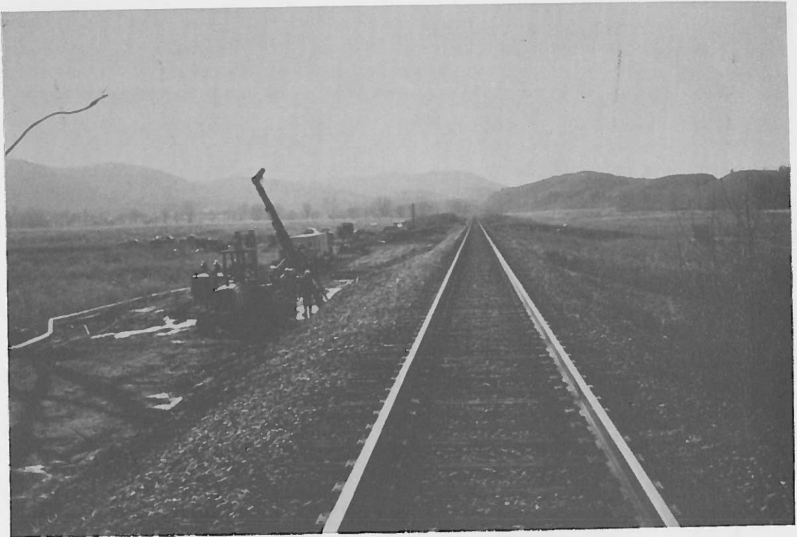
Figure 6. Photograph Facing Railroad South Showing Angle-Drilling Operations.
