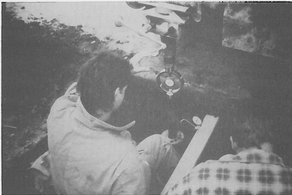
FIGURE 3 Conducting field CBSs on subgrade.
