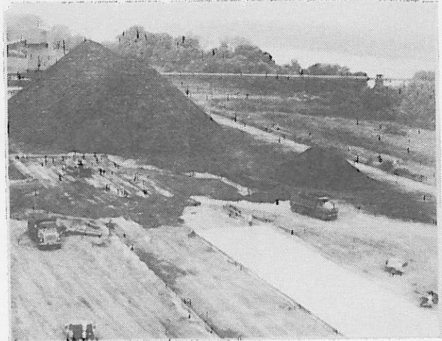
Figure 10. Photograph showing segmental pad repair activities
