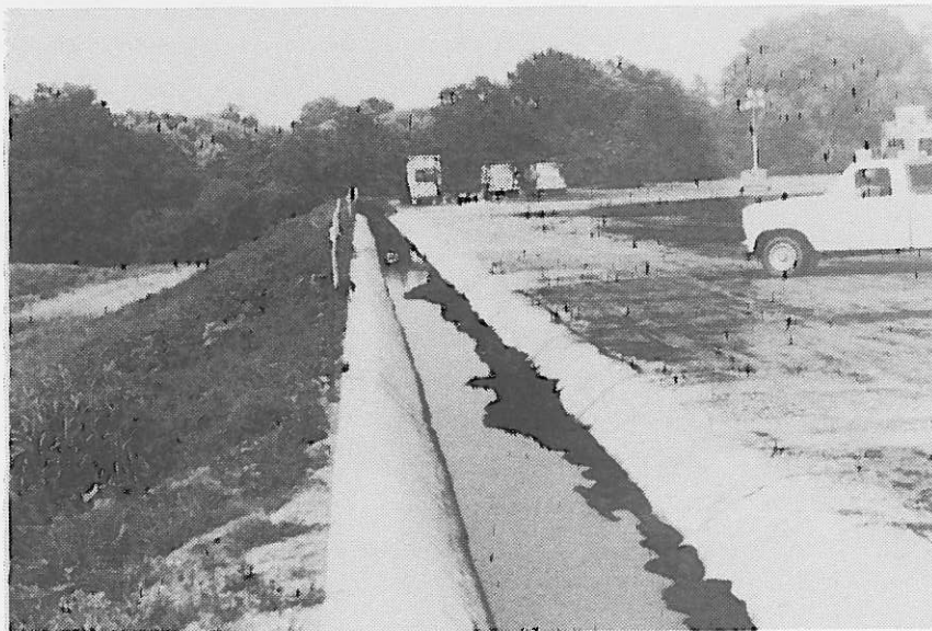
Figure 7. Photograph of reconstructed fill outslope and ditch
