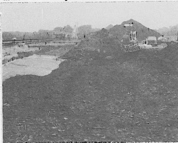
Figure 8. Photograph showing stabilization fabric and backfill within pad repair area
