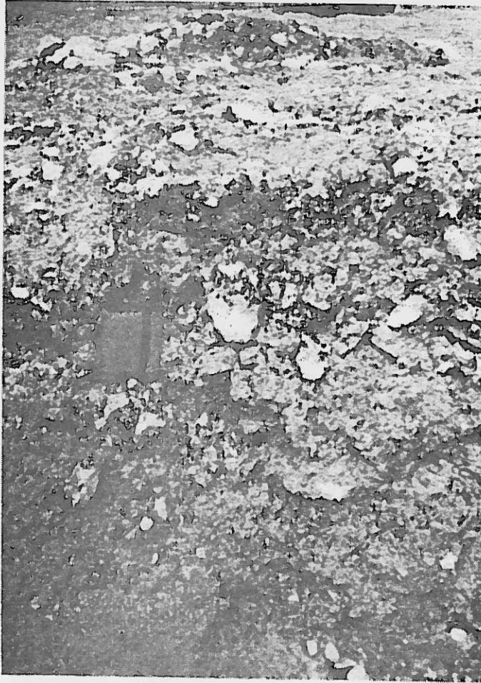
FIG. 1. Typical Exposure of Rock-Soil Fill; Wallet at Left in Photo is Approximately 3.5 in. (5.3 cm) Wide by 5 in. (7.7 cm) High
