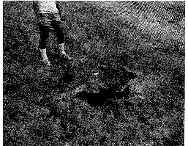
FIG. 10. Groundwater Exit Seep in Toe Area of Slide.
