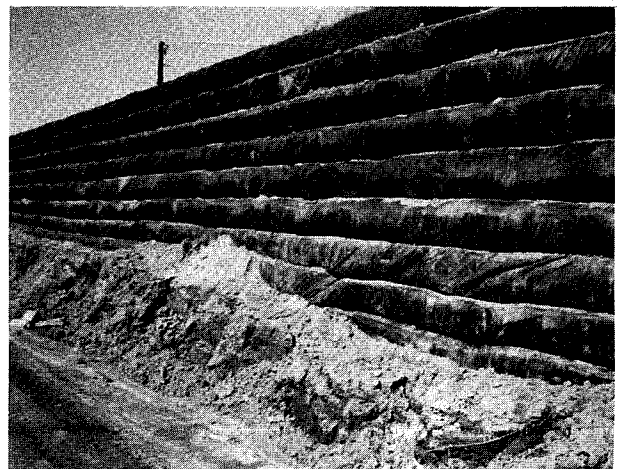
Figure 5. Completed section of the fabric reinforced wall.
