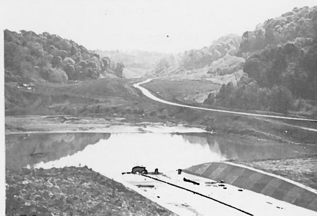
Figure 2. Slurry impoundment prior to current construction. Slurry line discharge is at rear of impoundment with pond next to embankment (Site 1).
