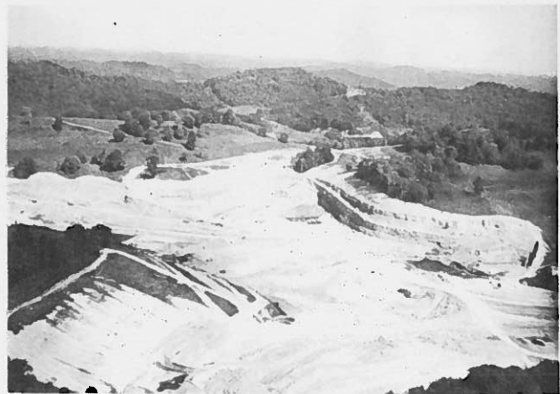
Figure 5. Strip mining and embankment construction operation (Site II).
