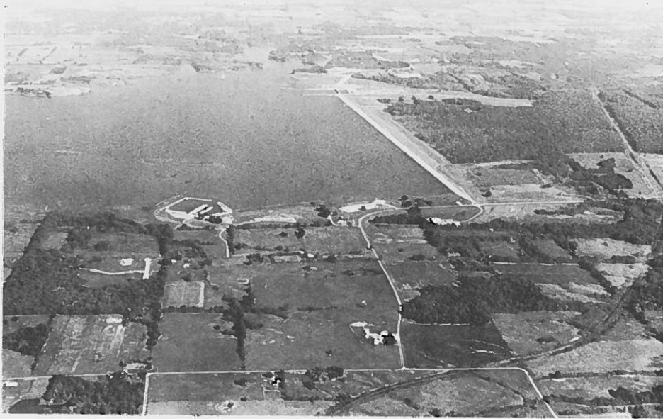
Figure 2. Oblique air photograph of Rend Lake dam and appurtenances, looking east.
